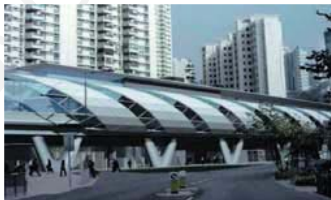
Figure 1.3.2.9 HAIDEP Light-rail Train
