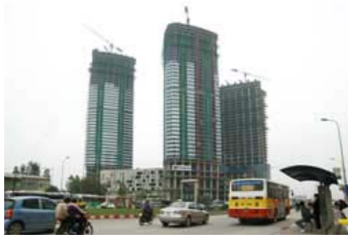
Figure 2.3.2.1 Keangram Landmark Towers
